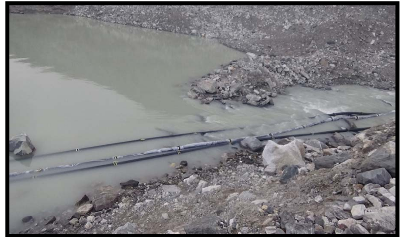
Siphoning of lake water using heavy duty HDPE pipes
