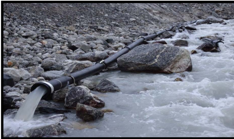
Siphoning of lake water using heavy duty HDPE pipes
